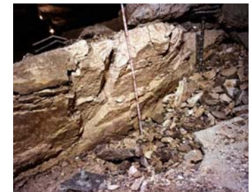
Explosion-driven floor drift in tuff, Nevada Test Site
