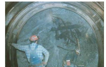
Effects of an uncontrolled cave in a block caving mine, CO Courtesy of F. Kendorski, 1976
