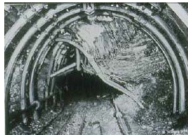
Effects of a bump in a coal mine, Belgium. Courtesy of P. Stassen, 1985.
