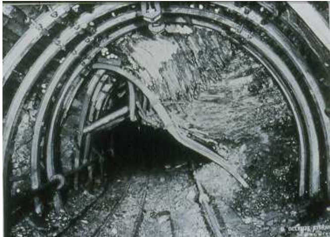
Effects of a bump in a coal mine, Belgium. Note the buckling of thin rock layers. Courtesy of P. Stassen, 1985.
