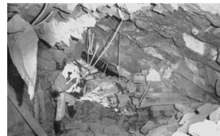
Effects of a rock burst in a South African gold mine Courtesy of D. Ortlepp, 2003
